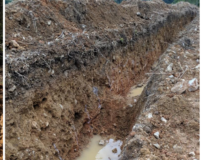
Trench 4 at Nanko (looking South)
